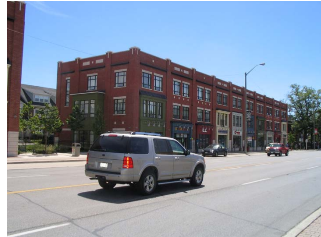
Example of new Live/Work development along Lakeshore Blvd (Port Credit)
