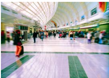
Pearson Airport – Terminal 3 Building
