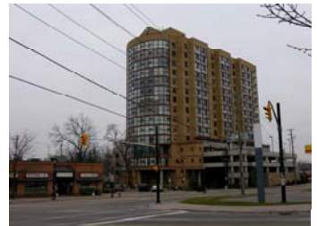
Church Street – Affordable Housing
