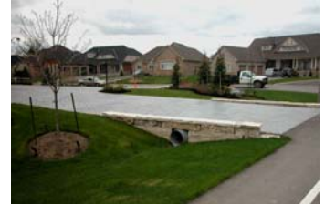
Springbrook Surface Run-off Treatment
