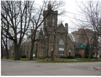
St Andrews Presbyterian - Church Street
