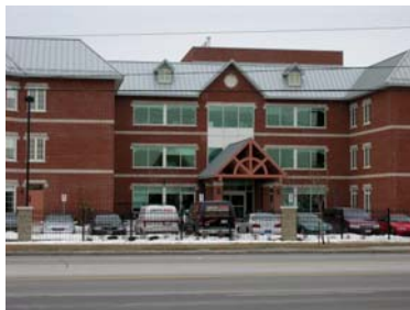
Woodhall Park Long Term Care Facility
