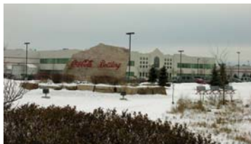
Coca-Cola Bottling Plant
