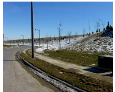
Torbram Road Noise Berm
