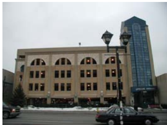
Example of Multi-storey Parking Structure
