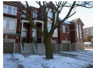
Infill Housing - McMurphy Ave N.
