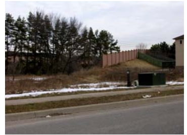
Residential Rail Noise Wall– Ravenscliffe Court
