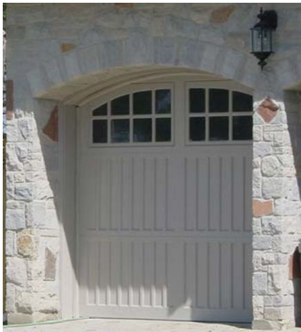
Fig. 3.3.1c - Image of recessed garage door
