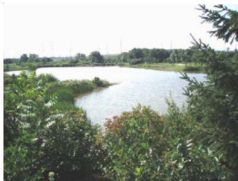
Fig. 2.9c - Existing Stormwater Management Pond
