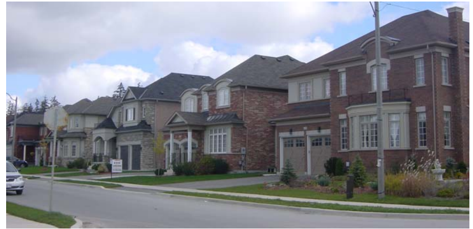
Fig. 3.1.3a - The street edge should be well-defined through building placement (Photo from "Streetsville Glen")
