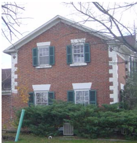
Fig. 3.2.1a - The Georgian architecture of Levi Hall House should influence the architectural style for new housing in Streetsville Glen West
