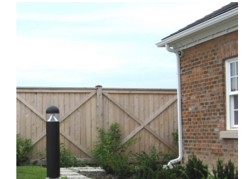
Fig. 2.4c- Heritage Fence Condition
