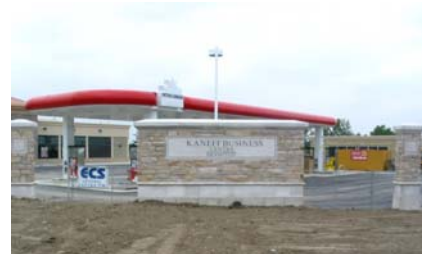
Fig 2.3e - (B) Feature at Mississauga Road & Hallstone Road, (C) Feature will be the same
