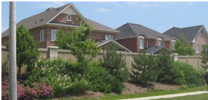
Fig. 3.1.1f - Image of existing reverse frontage dwellings on Financial Drive (Photo from Hallstone Road - "Streetsville Glen")
