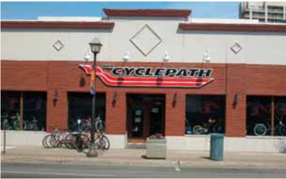
Downtown façade improvements program
