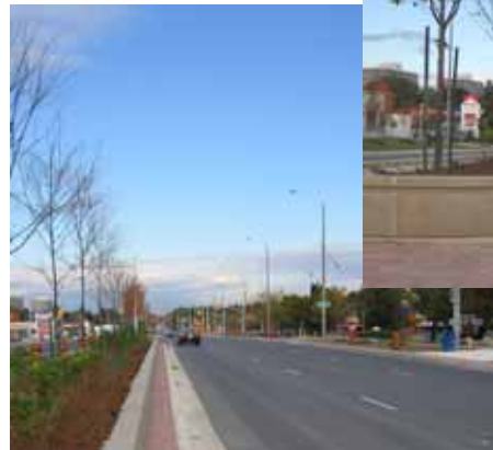
South Gateway streetscape improvements (Main and Steeles)
