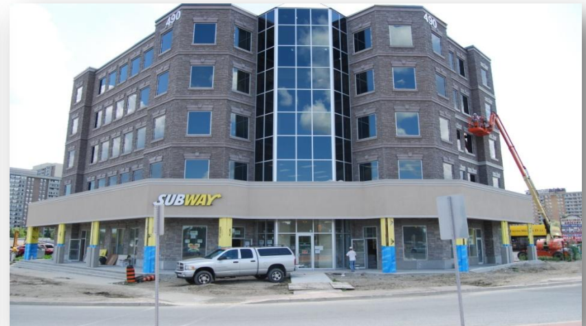
RE/ MAX BUILDING – 490 Bramalea Road
