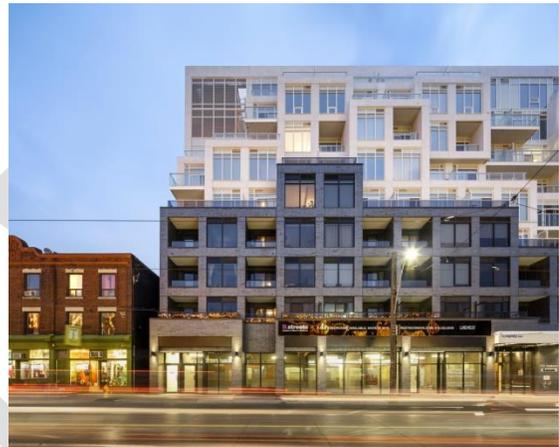
**Figure 12 Mid-Rise Building with Stepback to Match Street Wall**
