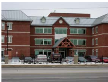
Woodhall Park Long Term Care Facility
