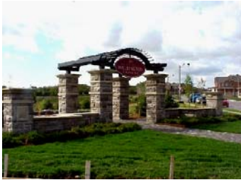
Springdale Entry Feature
