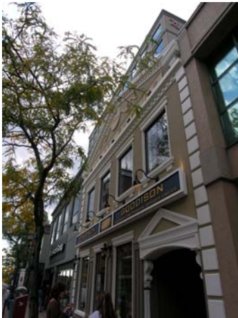
Building Façade Improvements
