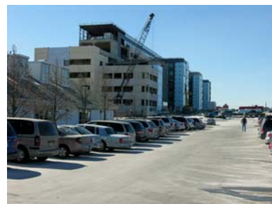
William Osler Health Care Centre – New facility under construction
