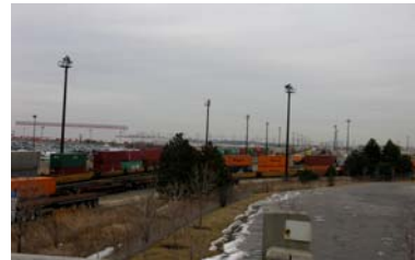
Brampton CN Intermodal Terminal
