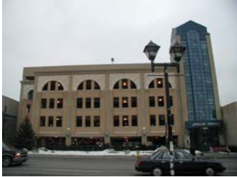
Example of Multi-storey Parking Structure
