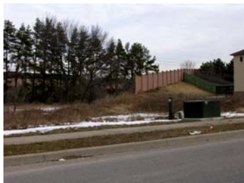
Residential Rail Noise Wall– Ravenscliffe Court
