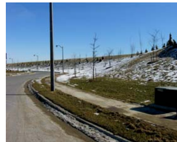
Torbram Road Noise Berm
