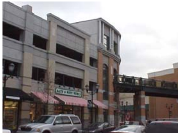
Parking Structure with Retail at the Main Level
