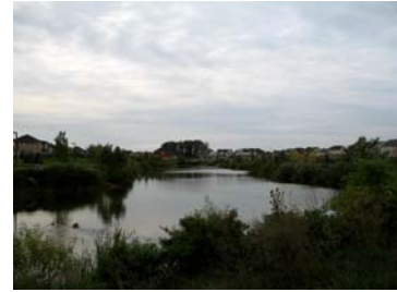
Hulme McClure Stormwater Management Pond
