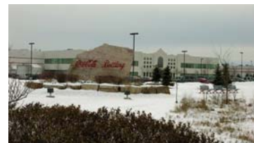
Coca-Cola Bottling Plant
