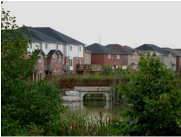
McClure Channel – Opportunity for Stormwater Recharge
