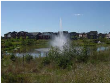
Danimar Stormwater Management Pond
