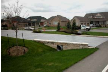
Springbrook Surface Run-off Treatment
