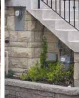
Utility meters screened, recessed and integrated into the townhouse design
