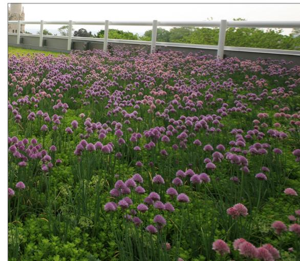
FIGURE 54 - Vegetated roofs minimize surface run-off .
