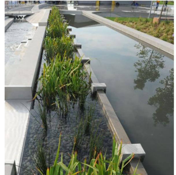
FIGURE 14 - Bio-retention water feature.
