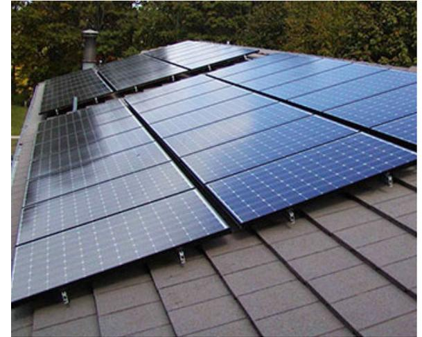
FIGURE 13 - Roof mounted photovoltaic system.
