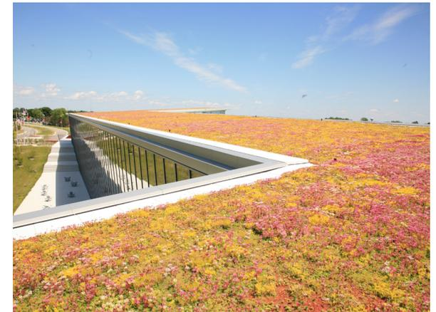
FIGURE 92 - A green roof minimizes surface run-off and reduces urban heat island effect.
