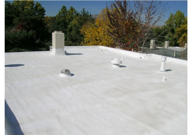
*FIGURE 93 - Light coloured roofs have a high solar reflectance, which reduces energy costs and reduces urban heat island effect.*
