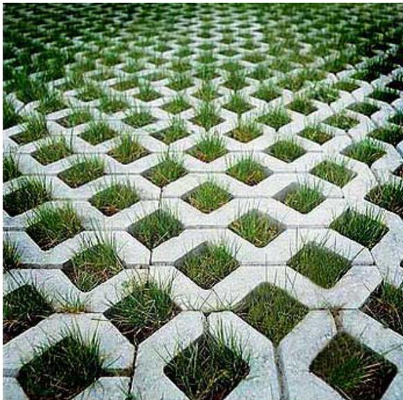
FIGURE 50 - Pervious surfaces that allow water to soak into the ground.
