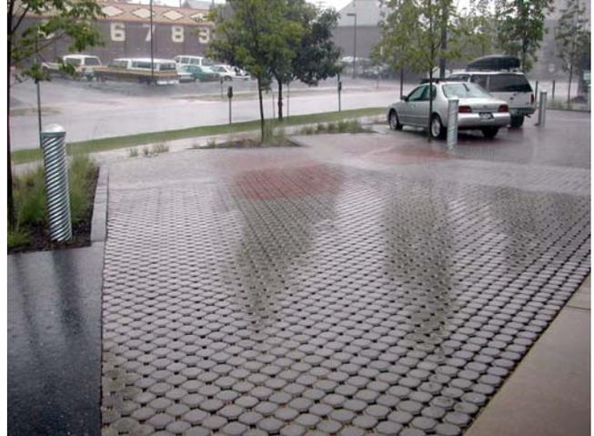
**Figure 2.1 - Permeable Paving**
