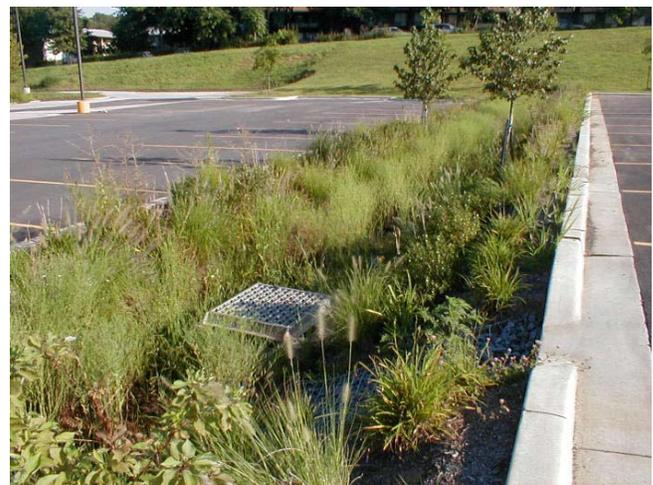
**Figure 2.2 - Bioswale**
