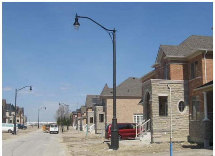
**Figure 5.27 - City of Brampton new standard Luminaire and Pole**
