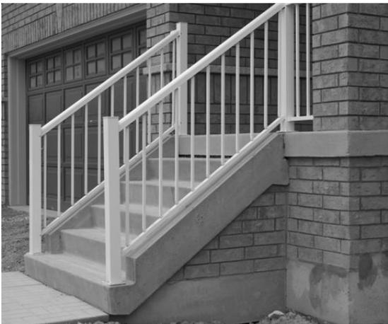
Figure 3.5a: Acceptible Precast Step Solution
