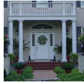
Figure 3.2.3.5.5a - The Main Entry Should Be A Focal Feature of the Home
