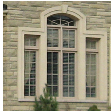
Figure 3.2.3.5.10a - Example of Coloured Window Frames
