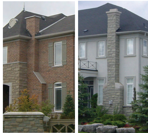
Figure 3.2.3.5.4d - Images of Corner Lot Dwellings With Chimney
