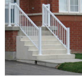
Figure 3.2.3.5.5b - Precast Steps Are Not Permitted At The Main Entry
