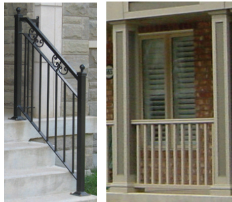
Figure 3.2.3.5.5e - Railings Should Suit the Style of the Dwelling
