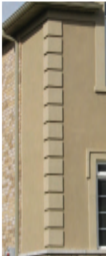
Figure 3.2.3.5.4b - Correct Application of Stucco Quoining (Even Spacing)
