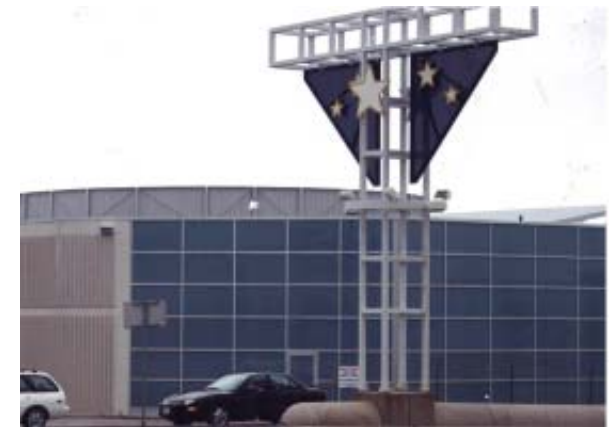
Roof Top Screening
