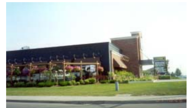
Landscaping at Site Edges
