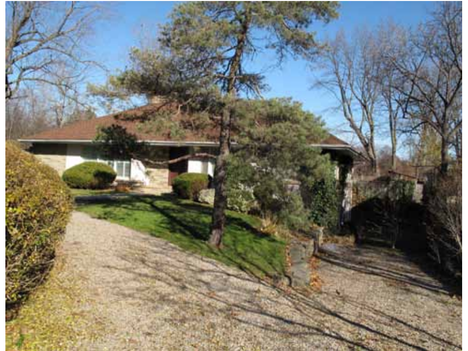
68 Main Street S, constructed in post-war period, Ranch Style.
