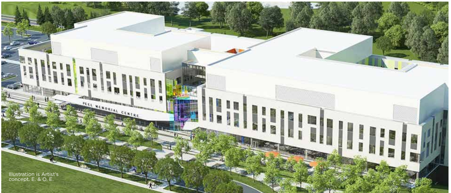
Peel Memorial Phase II expansion
